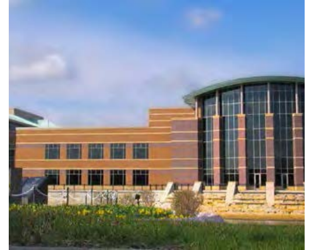
DuPage County Courthouse
