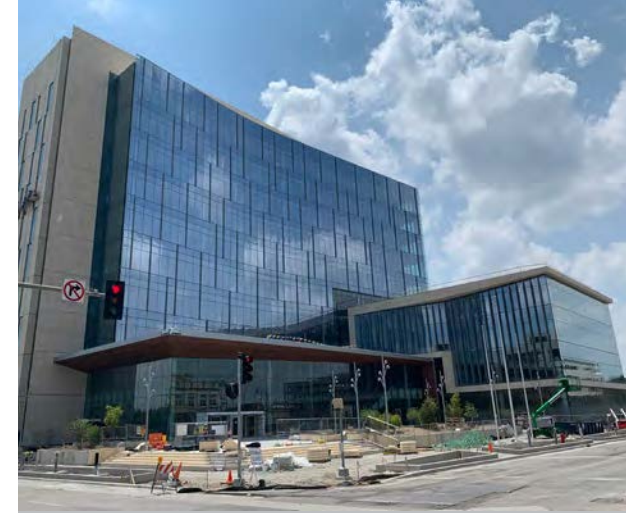
Will County Courthouse
