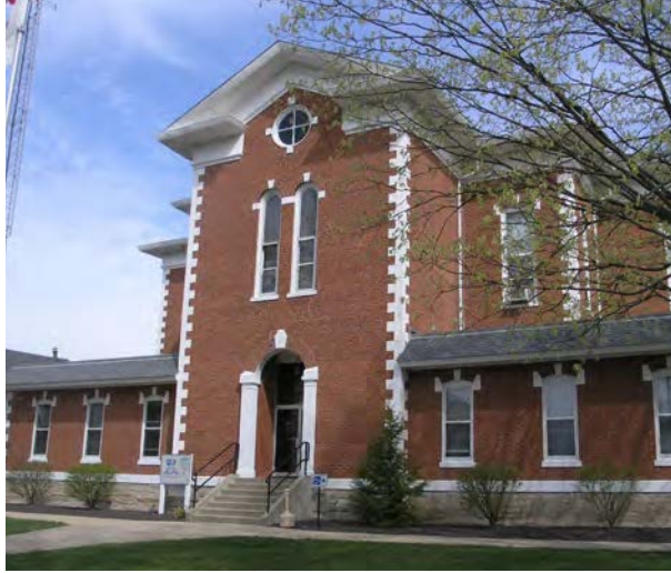
Washington County Courthouse
